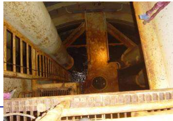
Risers inside steel caissons
